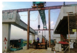
PC Super-T Girder Launching
