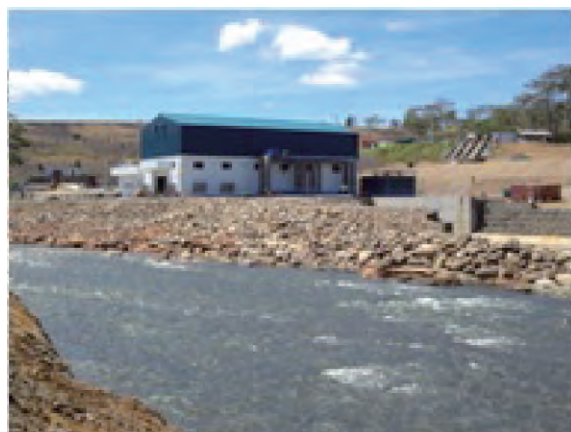
Bolder riprap against flooding
