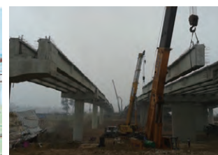
I-Girder Erection at Ca Lo Bridge
