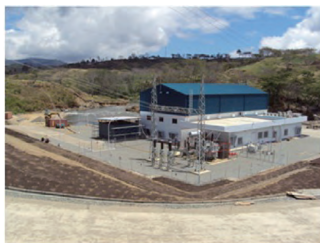
Outdoor switchyard & transformer
