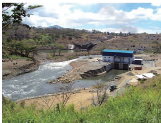
YTOD power station & tailrace channel
